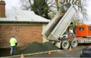
Toilet Construction commenced
